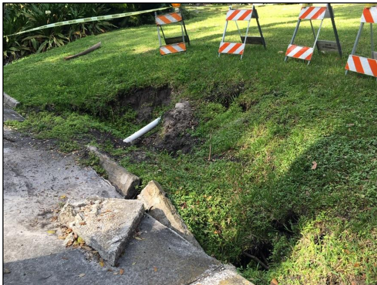
Figure 1: Ground erosion near where the art installation was to be located.
